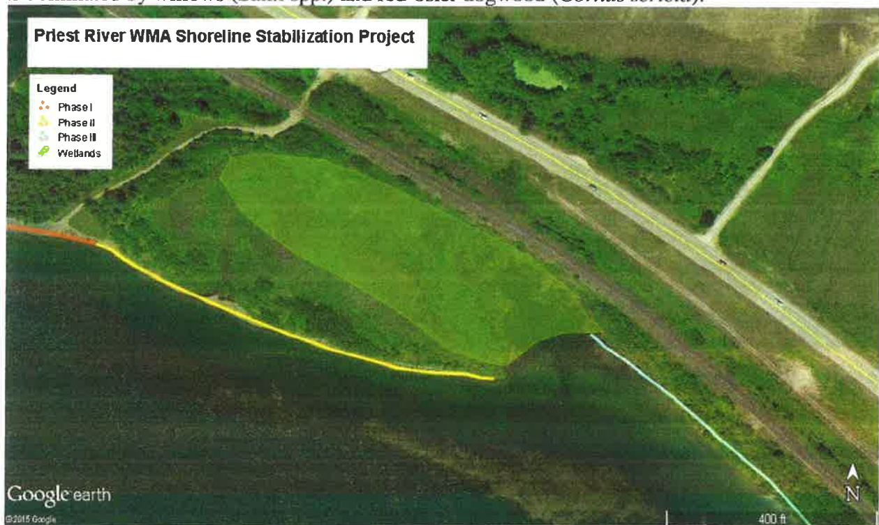
Figure 4. Wetlands adjacent to shoreline stabilization projects
